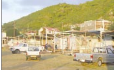
Work going on at Carnival Village in Marigot.
