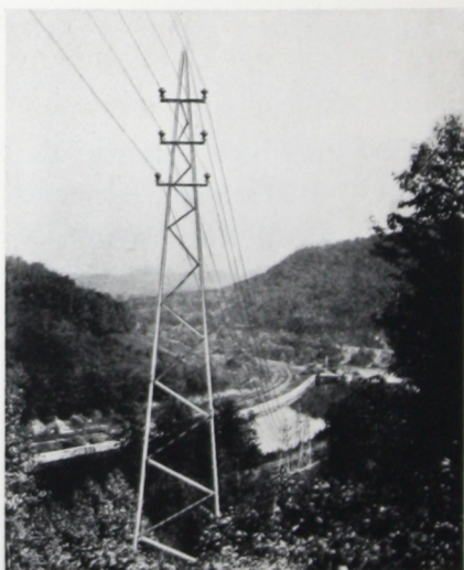
Flexible "A" Frame Transmission Tower Line, Built for Eastern Pennsylvania Power Co.
