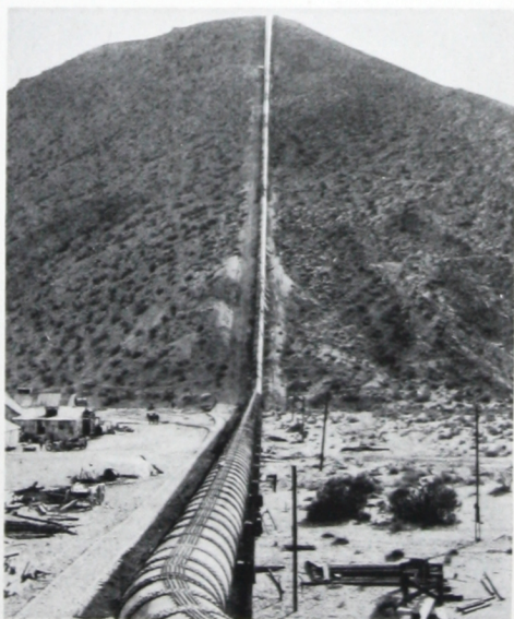
10' 0" Diam. Penstock—Jawbone Canyon Syphon, City of Los Angeles, Cal.
