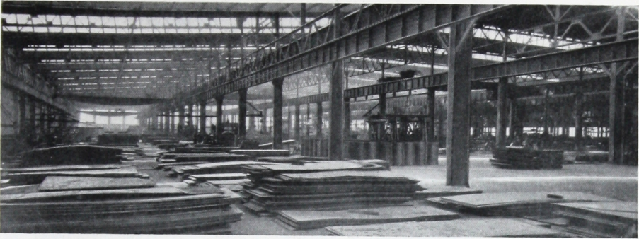
Partial Interior View of Riter-Conley Shop No. 1
