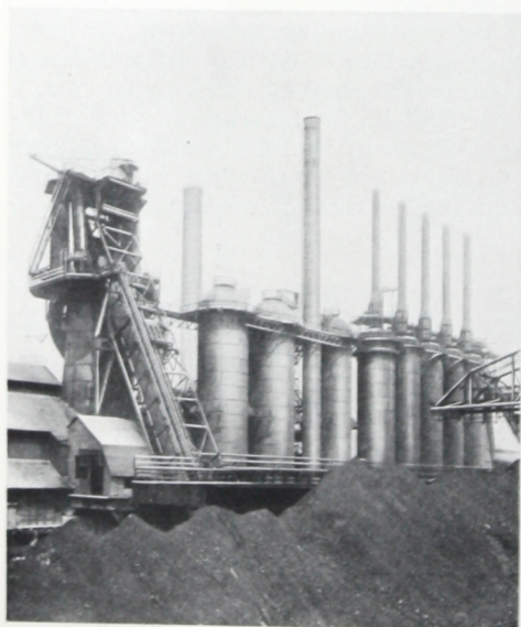
600-Ton Blast Furnace Built for Pittsburgh Crucible Steel Company Midland, Pa.
